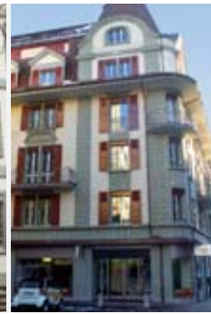
Energie Wasser Bern (ewb), Bern
