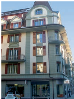
Energie Wasser Bern (ewb), Bern
