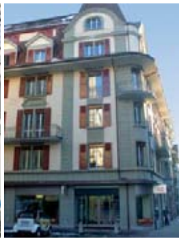
Energie Wasser Bern (ewb), Bern
